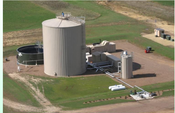
Five Star Dairy Facility - Elk Mound, WI
