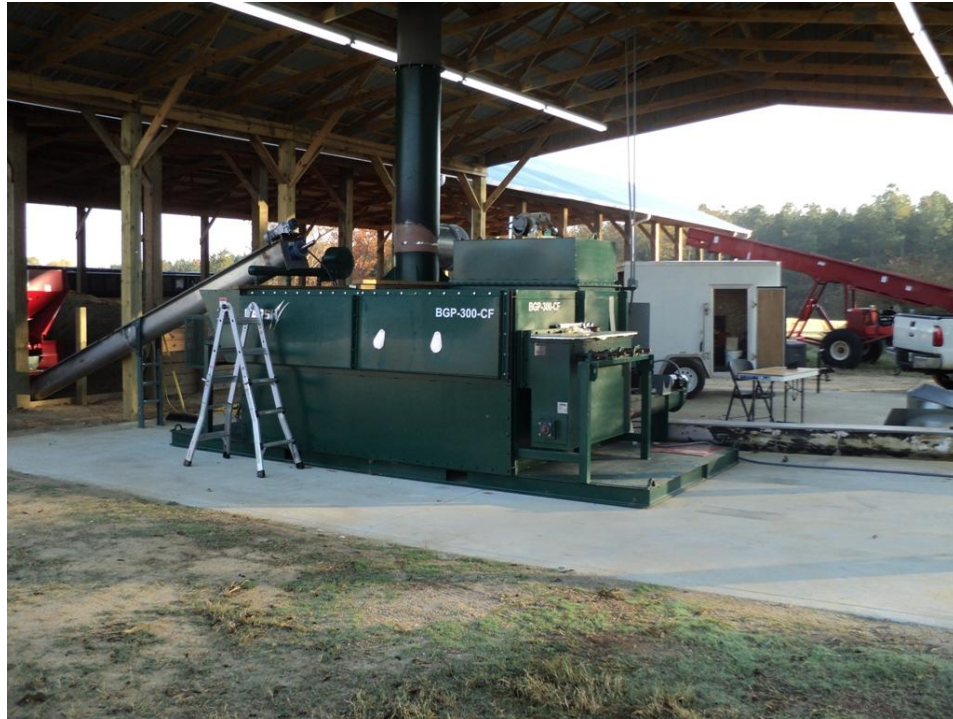
Figure 2 –gasifier feed system being installed
